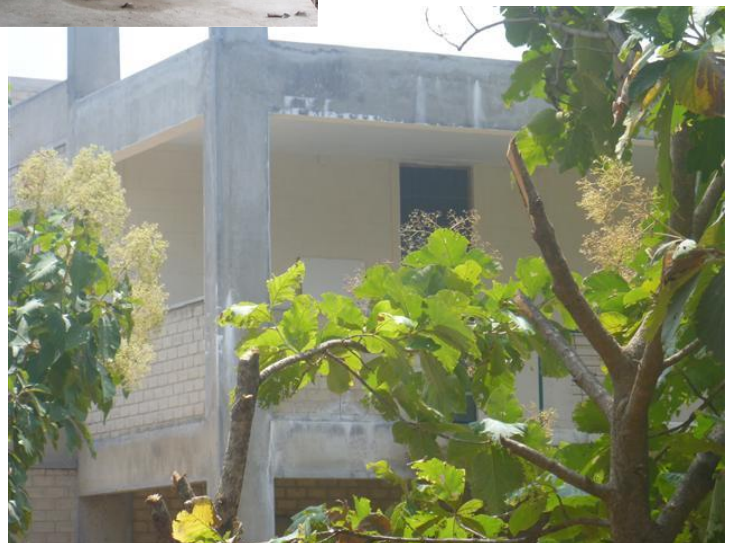
The front balcony... nearly completed!
